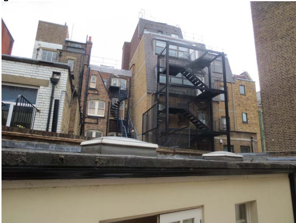
View looking south-east towards the rear of Bond House
